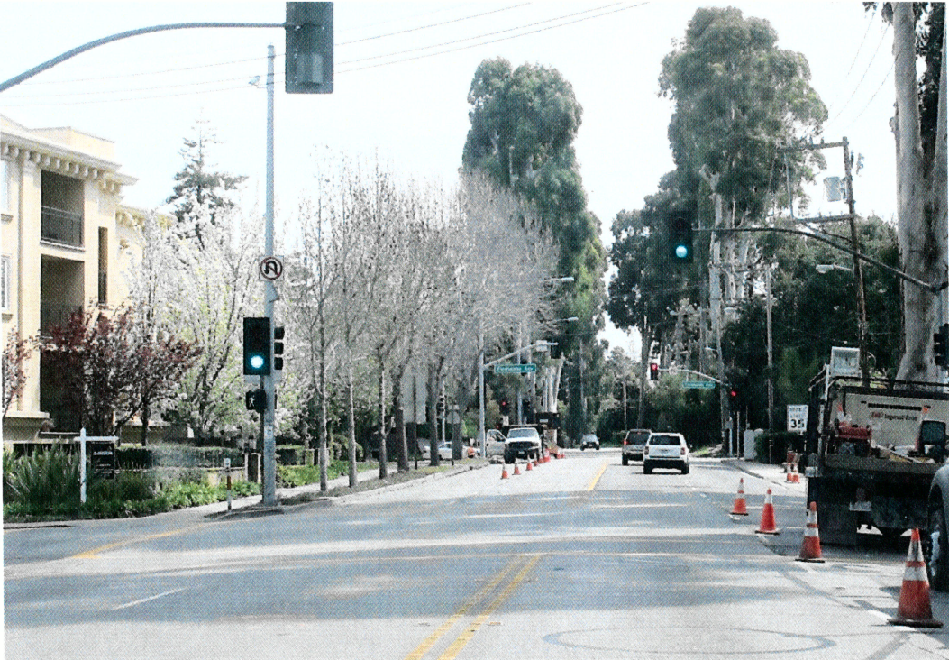
Existing view from Oak Grove Blvd and El Camino Real looking South
