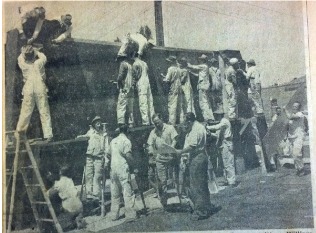
CARPENTRY WORK on Burlingame's Honor Roll nears completion on the Park Road lawn of the post office as more than 30 volunteers aided in the construction last Sunday morning. Shown in front of the roll, consulting plans, are left to right, U. S. Simonds Jr., business agent of Carpenters Local 162 and chairman of the construction committee; William Feary, member of the construction committee, and George McQueen, who serves on the general committee of which Emil Schultz is chairman. Plastering work on the roll is expected to be done this weekend and work has started on painting the names of the servicemen and women on the panels. (Photo by Anita Fowler).
